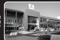
Instrument Transformers Unit Hosur
