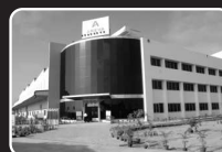
High Voltage Switchgear Units Padappal
